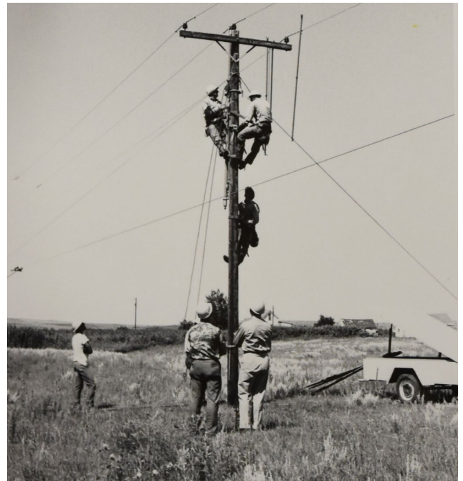
Lineworkers electrify KEM Electric's power lines in 1962.
