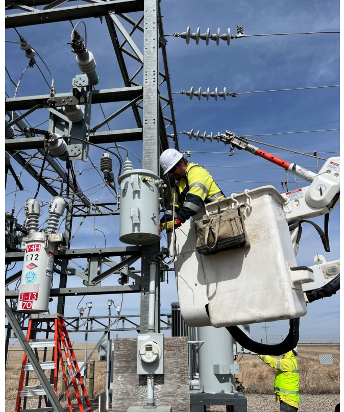
Austin Ohlhauser , journeyman lineworker works to install a new transformer in the Danzig Substation.
